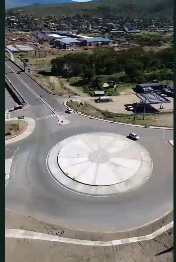
100 year old Single lane Steelbridge Refurbishment New 4 lane Concrete Bridge over Steelpoort River
